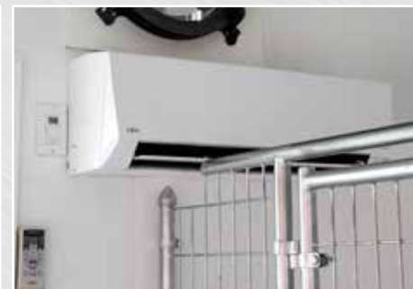
Interior View of Mini Split Heater/AC Unit
