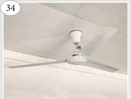
110 volt Ceiling Fan with reversible variable speed switch, 27,000 CFM
