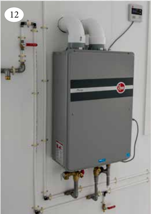
On Demand Water Heater Uses LP and Electric
