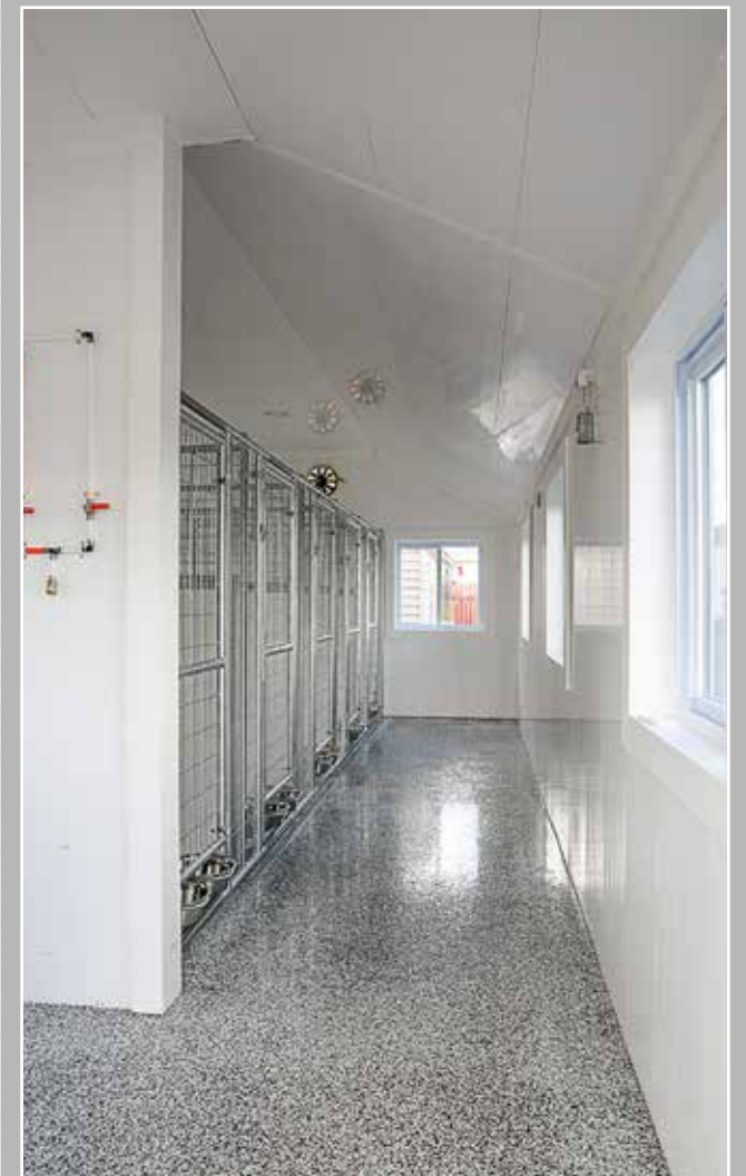
Interior View Of 10x28 5 Run kennel with 3' overhang with 10' Add on runs. Showing welded wire panels and exhaust fan.
